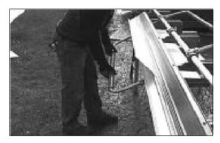
Figure 5-2 Hand and On-Site Tools Limit Panel Size
