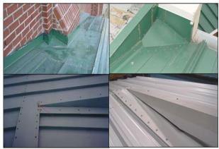
Figure 19-14 Roof to Wall Flashings Vary Widely
