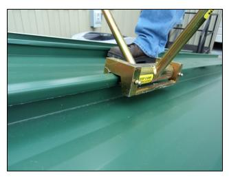
Figure 12-10 Hand-Seamer/Crimper
