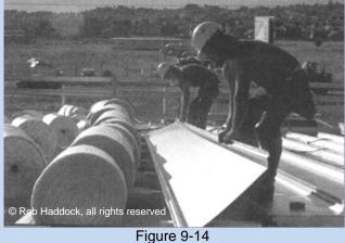
Proper Lifting Of a Roof Panel
