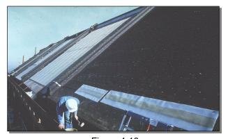
Figure 4-18 Solid Substrate, with Underlayment, For Installation of an Architectural Panel Roof
