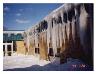
Figure 10-22 Undesirable Ice, Icicles, and Ice Dams
