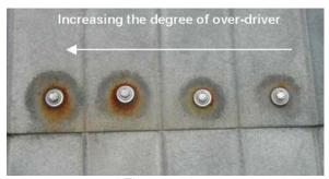
Figure 10-79 Over-Driven Fasteners
