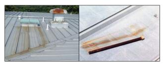
Figure 10-41 Corrosion Damage to a Metal Roof
