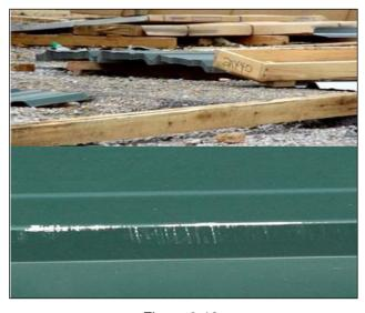
Figure 9-12 Improper Staging of Material Will Cause Damage
