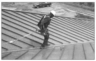
Figure 9-3 A Personal Fall-Arrest System (PFA) Includes a Harness, Lanyard, and Anchor System
