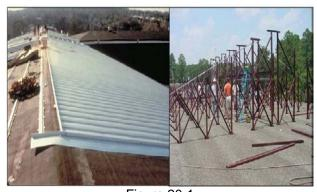
Figure 20-1 Two Re-Covering Methods Metal Overlay (Left) and Retrofit (Right)
