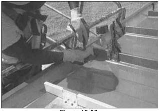
Figure 16-28 Spacer Tools Help Hold Panel Module
