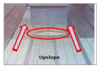
Figure 8-8 A Properly Designed and Installed Curb Note Cricket and Drainage Clearances
