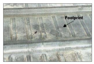
Figure 9-8 Inattention to Footwear May Cause Panel Damage
