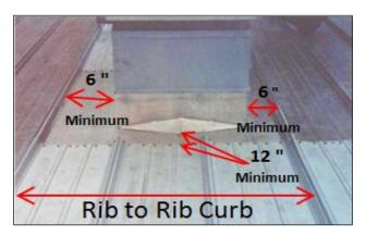
Figure 8-12 Recommended Curb Clearances
