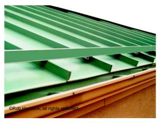
Figure 8-20 A Snow Fence Type Clamp Attached to Standing Seams
