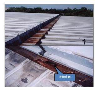
Figure 10-59 Incompatible Gutter, Flashing, and Roof Material
