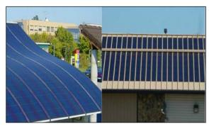
Figure 8-34 Photovoltaic Laminate on a Metal Roof
