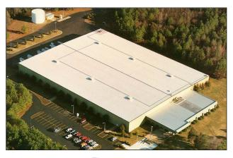
Figure 4-21 Hydrostatic, Low-Slope Roofs Must Address Slow-Moving Water Issues
