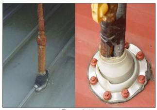
Figure 8-15 Incorrect Roof Jack Installation by Other Tradesmen
