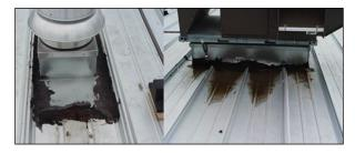
Figure 8-9 Improper Curb Types
