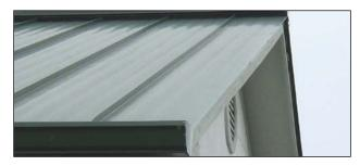
Figure 4-17 Architectural Panel Roof System
