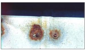
Figure 14-6 Incorrect Fastener Material Shortens Roof Life
