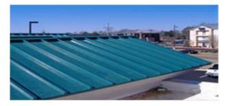
Figure 4-9 Modern Batten Style Roof
