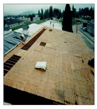
Figure 6-6 A Plywood Solid Roof Deck Substrate
