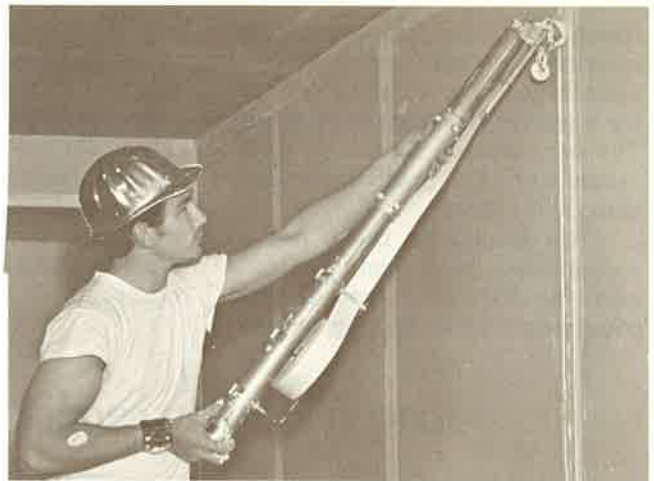
Fig. 50 Machine application of joint bedding compound and reinforcing tape.
