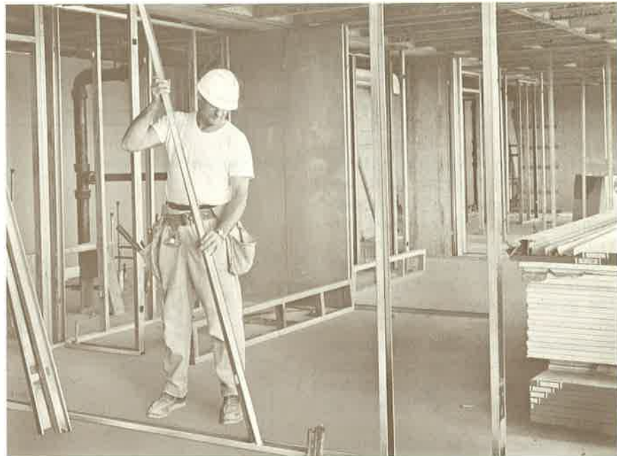
Fig. 18 Metal Studs go up quickly in this office building.
