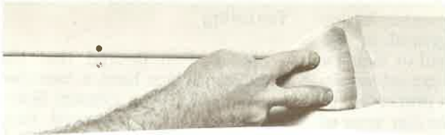
Fig. 47 Tape bedding compound being applied to tapered edges of wallboard joint.
