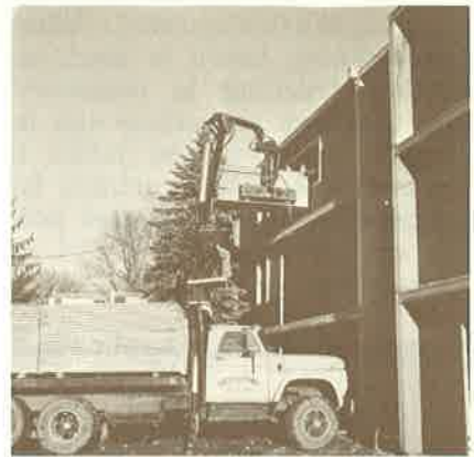
Fig. 9 A boom truck delivers gypsum board economically to upper stories.
