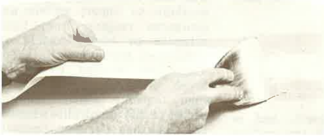
Fig. 48 Joint reinforcement tape being applied into bedding compound.
