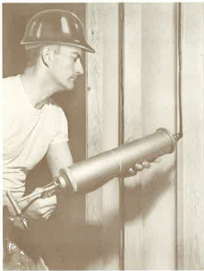
Fig. 25 Application with a stud adhesive gun.
