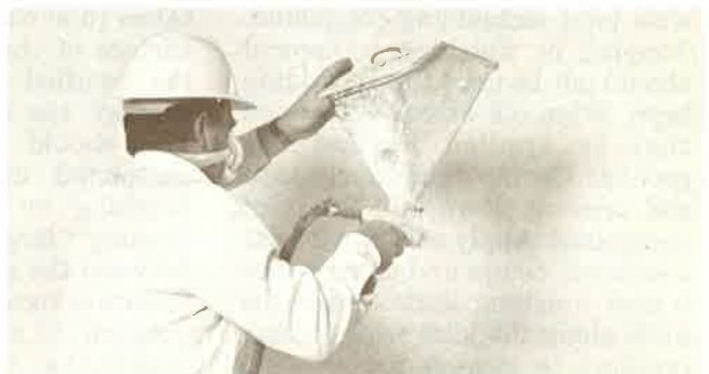
Fig. 51 A variety of textured appearances can be obtained by using a spray machine.
