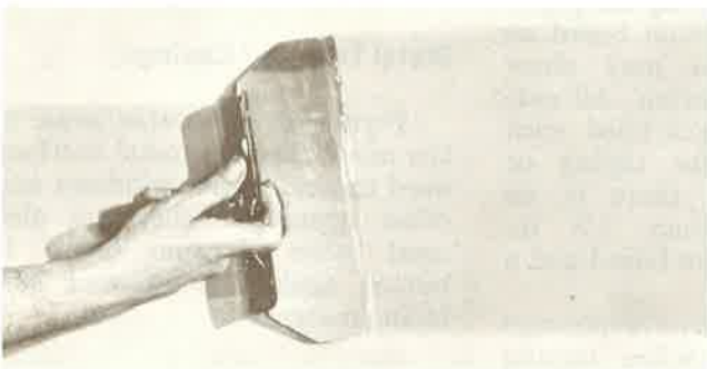
Fig. 49 Joint topping coats are applied.
