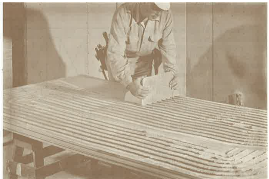
Fig. 38 Notched spreaders are used to apply adhesive for sheet lamination.
