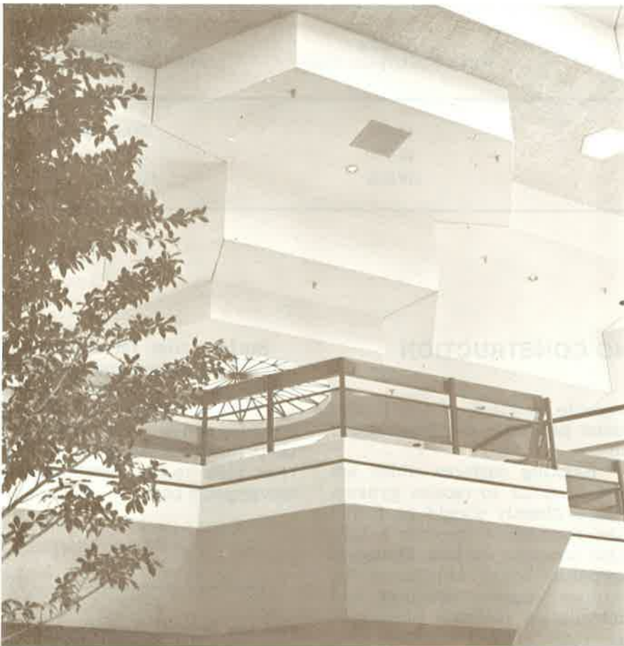
Fig. 45 Gypsum board walls and ceilings usually have joints treated with tape and compound to give a smooth, monolithic appearance.
